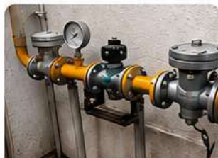
GAS REGULATION & METERING ASSEMBLY
