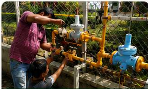
LPG PIPELINE INSTALLATION
